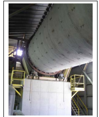
Pedestal foundation and access platforms for trunnion service
