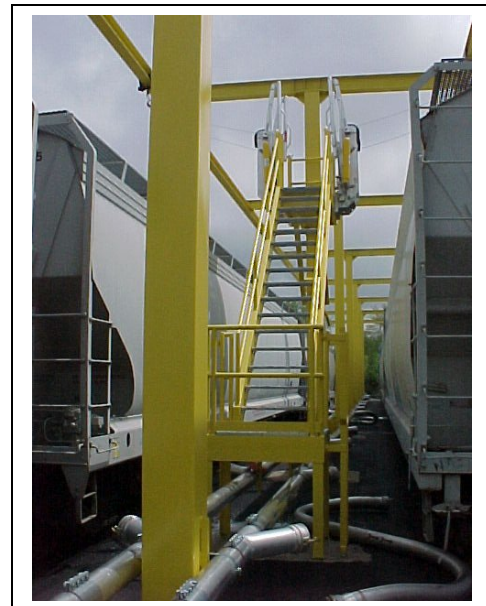
6" tubing manifold and fall protection system between the rail sidings
