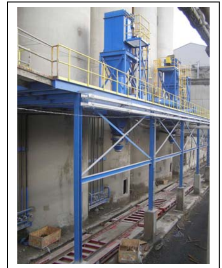
Overall view of structure supporting air slides and dust control equipment
