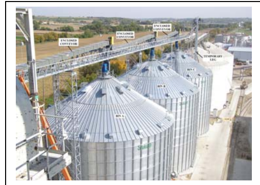
Three new bolted grain silos with closed feed conveyors
